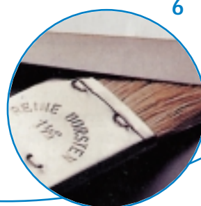
Longitudinal seam closed with special solvent-based adhesive
